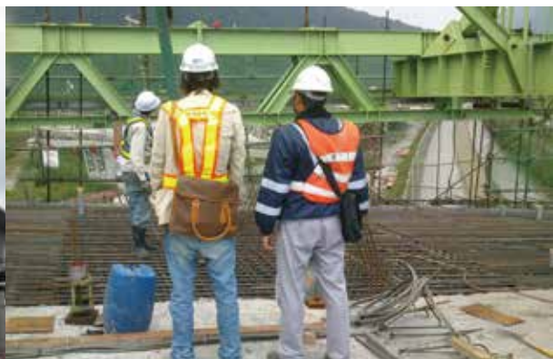
● P11施工全程監視
