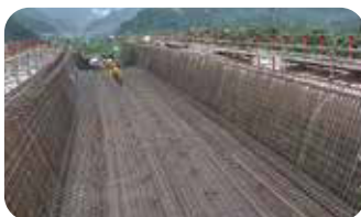
2.底、腹板鋼筋綁紮
