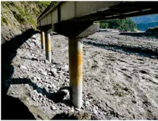
(a) 鋼橋墩柱及帽梁受洪流衝擊 (b) P7 橋墩防撞鋼板受洪流衝撞破損
