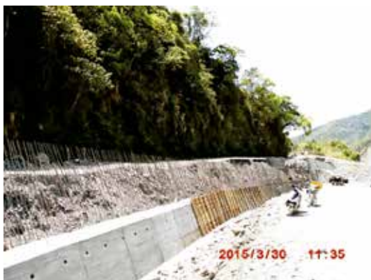
(c) 擋土牆牆身昇層施工
