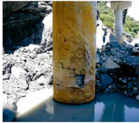
(a) 鋼橋墩柱及帽梁受洪流衝擊 (b) P7 橋墩防撞鋼板受洪流衝撞破損
