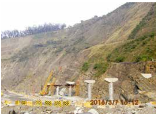
(c) P5~P7 帽梁施工
